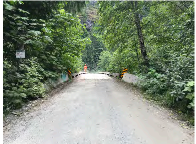
Approach from Right Bank when facing downstream
