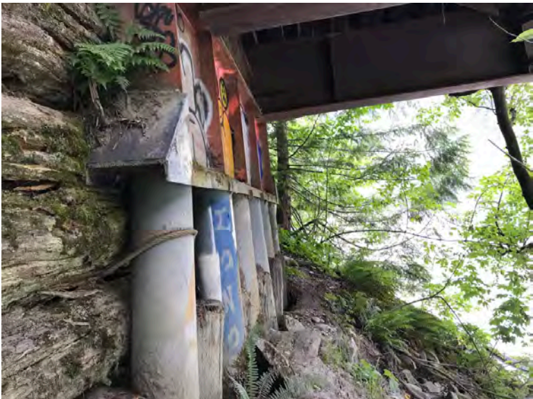
Right Bank Abutment when facing downstream
